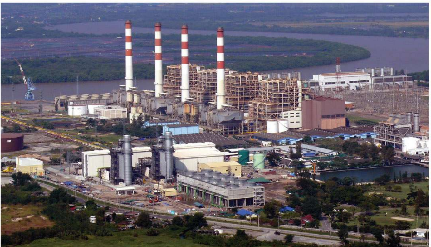
700MW Combined Cycle Power Plant, Bangkok, Thailand
